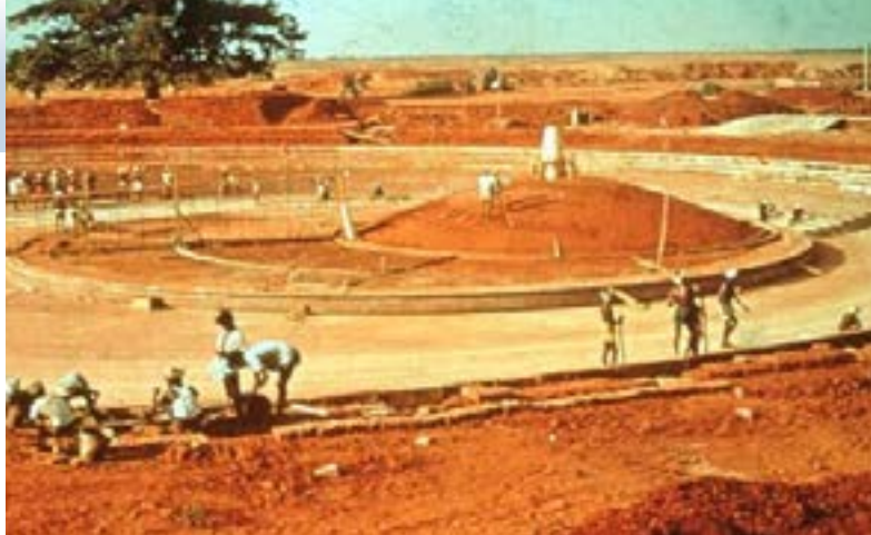
Construction of the Amphitheater
